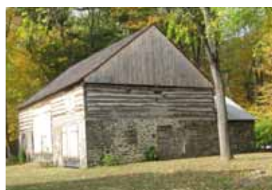
The Caruso barn is one of the very few ground barns where the lower halves of the exterior walls are stone and the upper halves are log.
